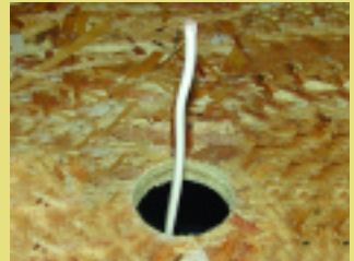
Figure 3 - Pull romex through floor.
