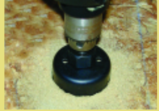
Figure 2 - Drill hole in floor using hole saw.
