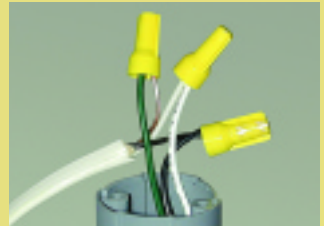
Figure 4 - Connect receptacle wires to romex. Be sure to match wire color(s).
