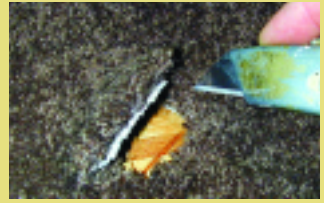
Figure 1 - Cut 2-3/8" hole through carpeting before using hole saw.
