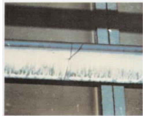
6 ENT™ secured to pipe above Blue Ballroom feeding four outlet and switch boxes in room. See Diagram I and Graph C.
