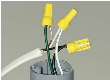
4. Connect receptacle wires to romex. Be sure to match wire color(s).
